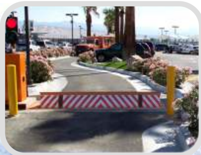
Security & Access Control
