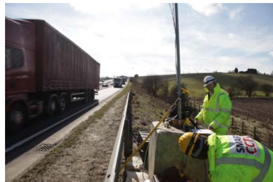
Installing a temporary video incident detection system for a traffic survey
